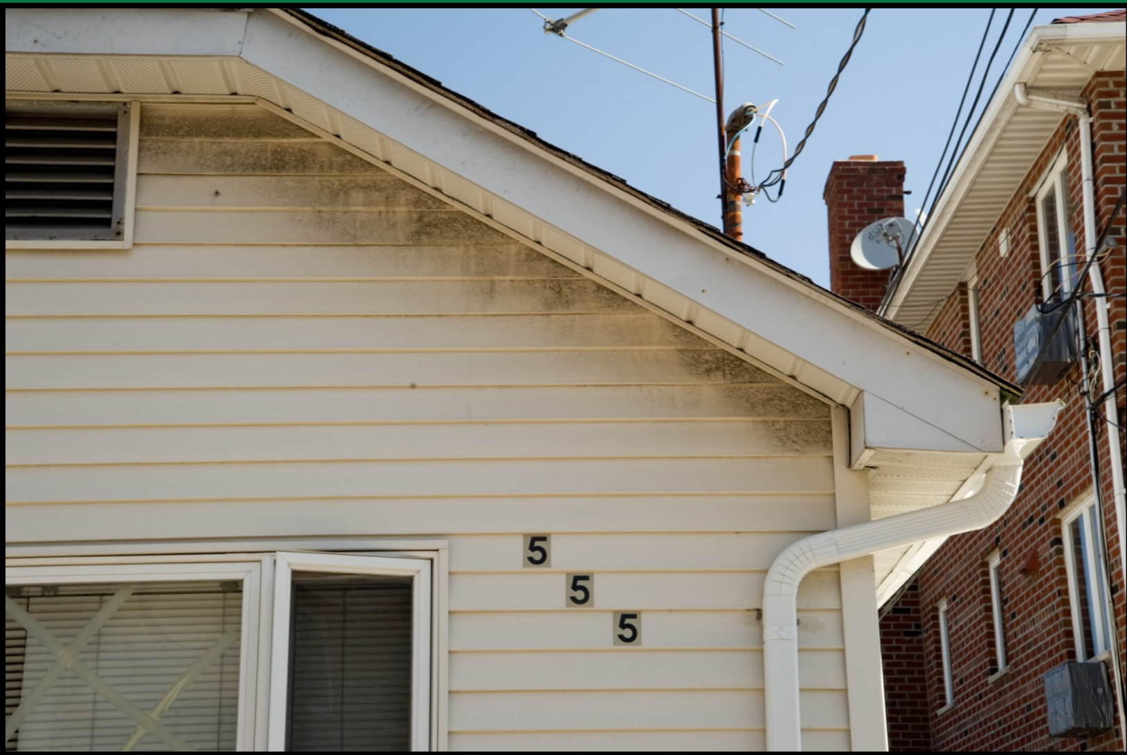
Mold on the exterior of home in Midland Beach. Photo: Karen Smul
