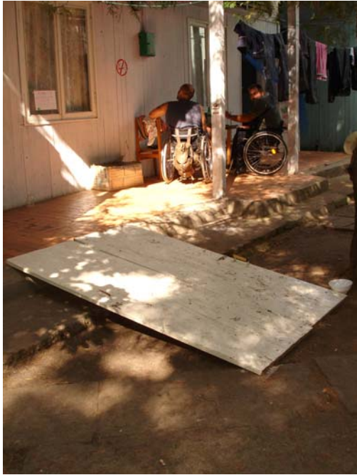
A makeshift wheelchair ramp
