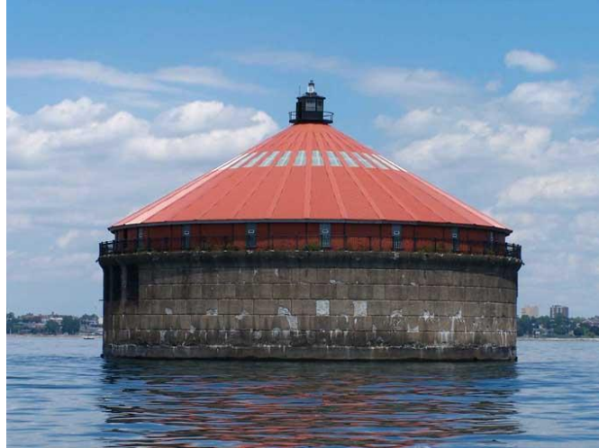
Water Intake Building, located on Buffalo's "Emerald Channel" 18
