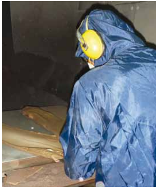
WORKER SANDBLASTING IN BANGLADESH. PHOTO: CCC GERMANY
